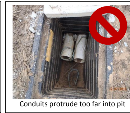
Conduits enter side (not end) of pit
