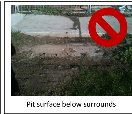
Pit installed in vehicular driveway
