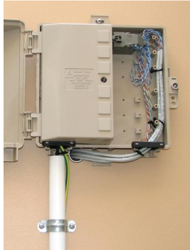
Cables running below the NTD
