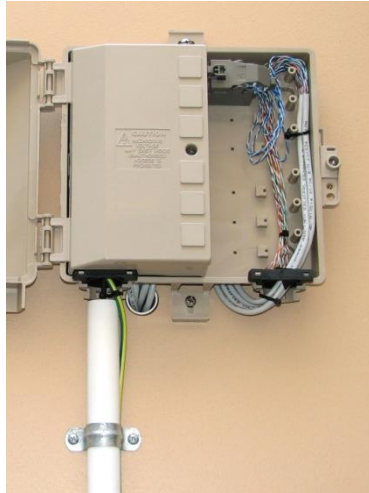
Cables running behind the NTD
