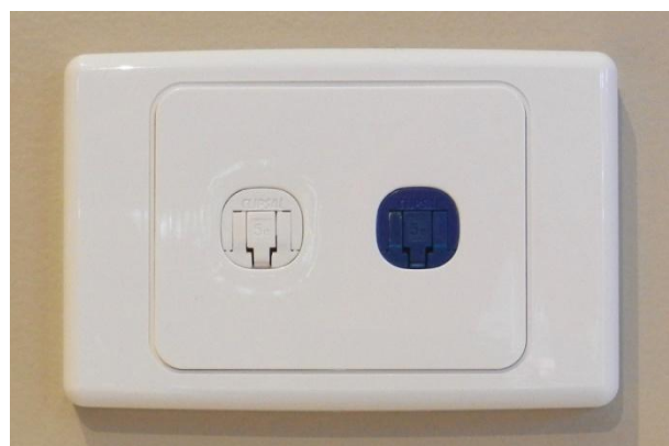
Figure 28 A typical TO with two colour-coded sockets
