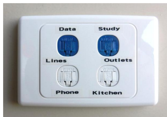
Figure 10 A typical multi-socket wall plate
