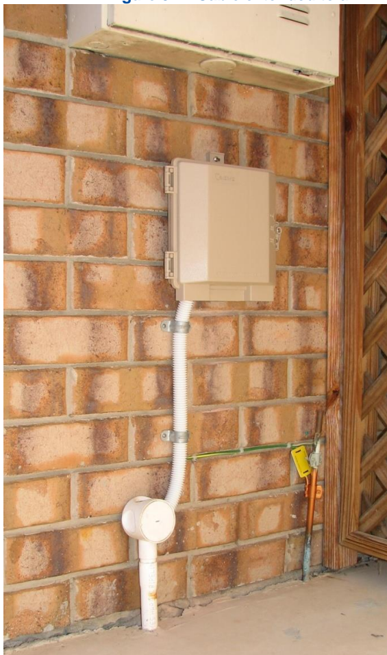
Figure 51 Cable extended to an NTD from an existing (obsolete) junction box
