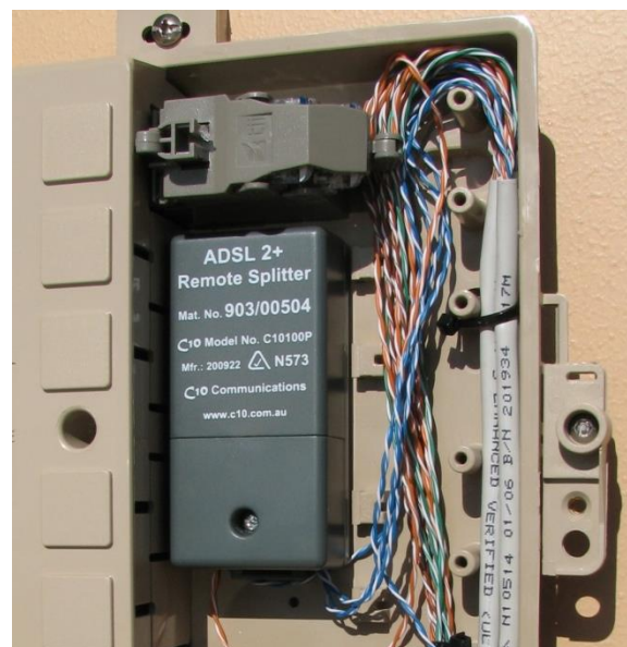
Figure 6 Central filter installed within a Telstra NTD (a) DSL line module (b) Filter in the customer compartment
