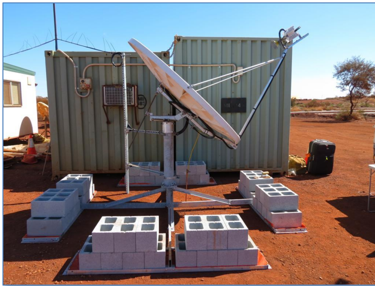
Figure 8: Besser Blocks only installed
