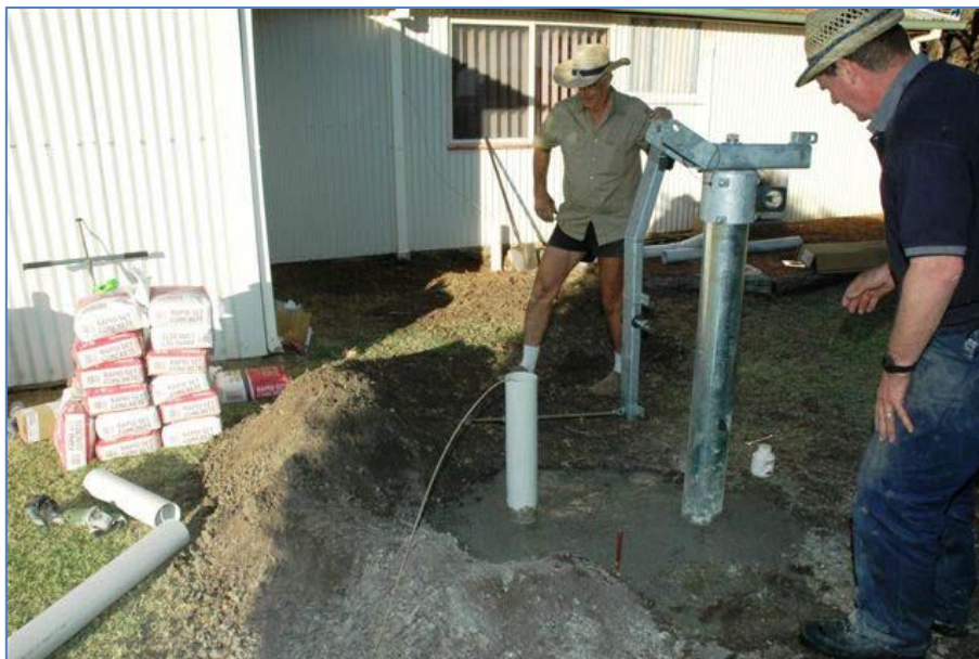
Figure 7: Post and Cable Run Riser installed
